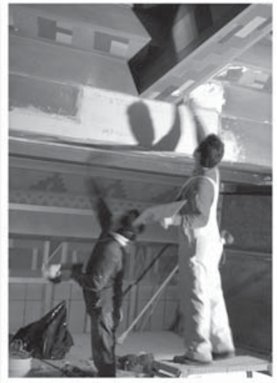
Painting the ceiling atop the Main Sanctuary
